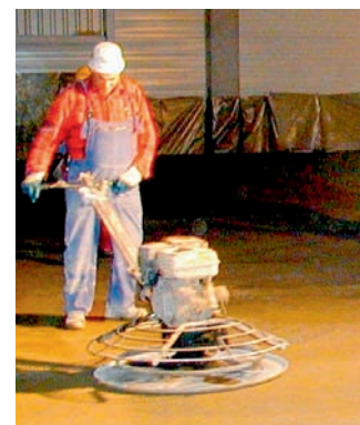
Concrete smoothing machine
