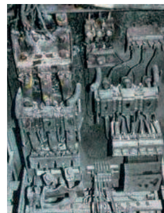
Control cabinet destroyed by fault arc
